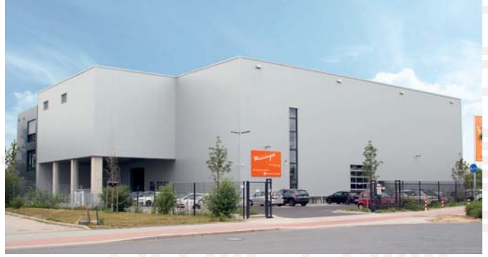
MEISINGER Headquarters Neuss, Germany
